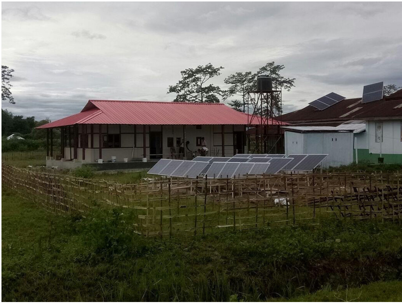
Figure 14.2 The modified KEBA sub-centre.
