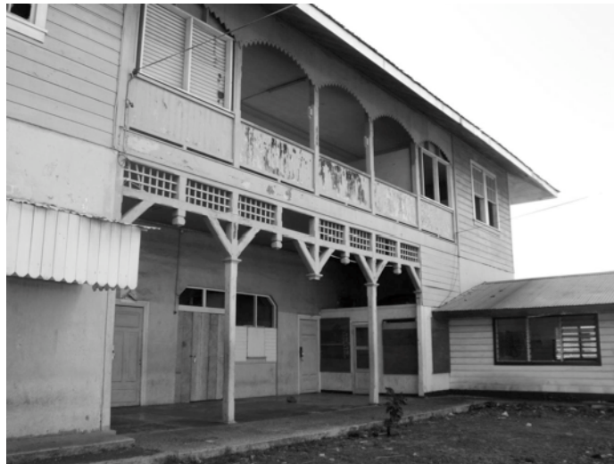
Figure 3 School Pavilion in Ifi-Ifi, Apia, before its conversion into the Museum of Apia, in 2006. Photo by author. Note the accentuation of the timber construction through chamfer and added knee braces.
