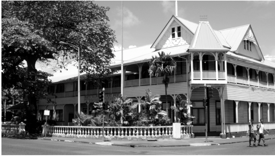
Figure 1 Court House, Apia. Built in 1903, extension in 1907 designed by Albert Schaaffhausen. Photo by author.
